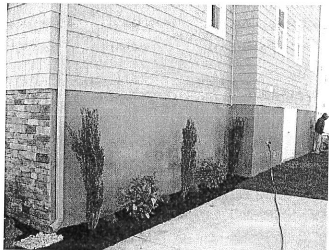
NORTH SIDE VIEW 11/13/2015
